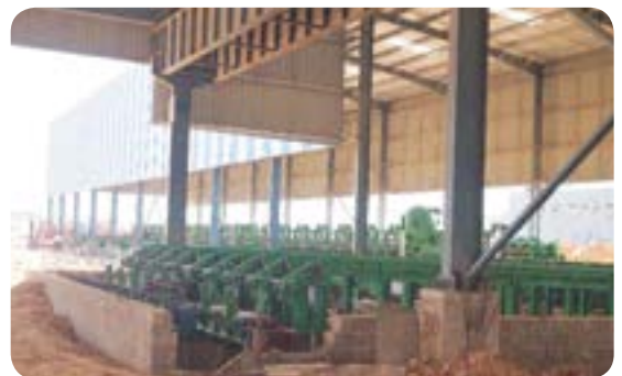
Equipment being installed in FABRIMETAL
